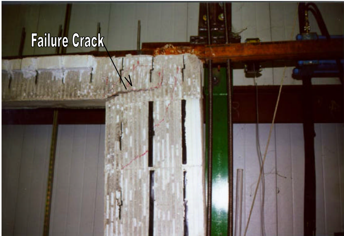
Figure 5 Failure Mechanism of Flat No. 3 Wall Specimen
